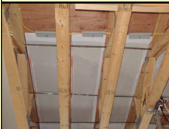
Ceiling Grid Heaters
